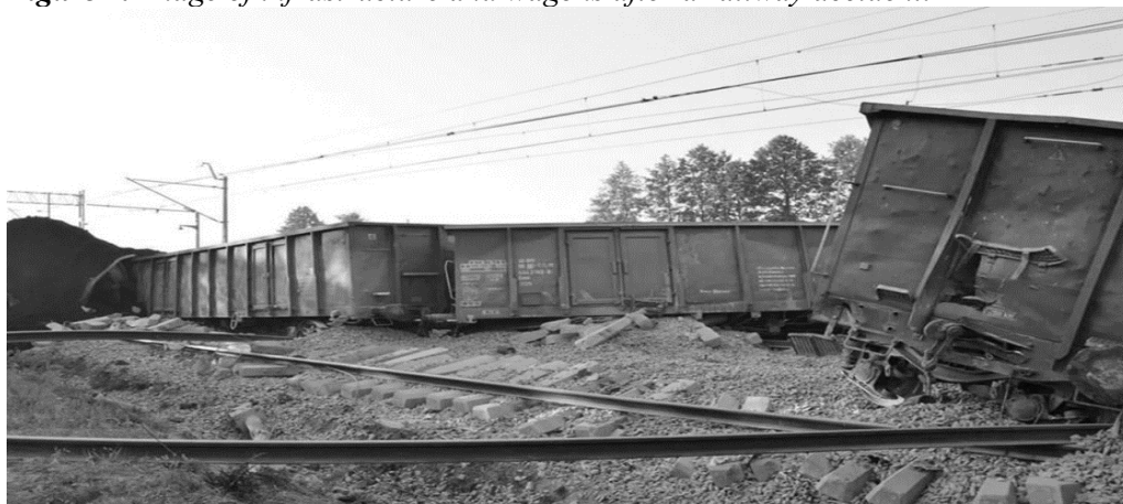
Figure 1. Image of infrastructure and wagons after a railway accident.
